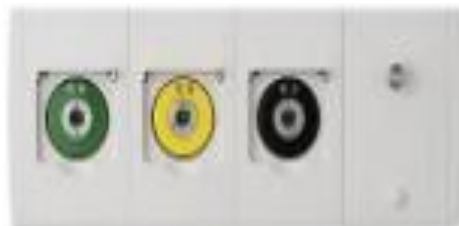
Embedded Type Outlet
